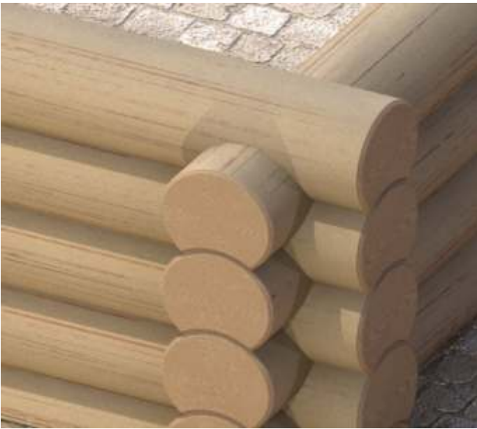
Flanged wall corner with moon shaped cuts and remains
